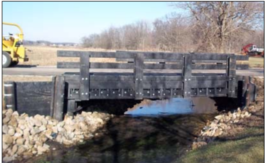
Bridge 174-0.56 over the Onion Ditch
